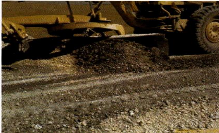
Figure 8: Field mixing of the studied base material with different steel slag content
